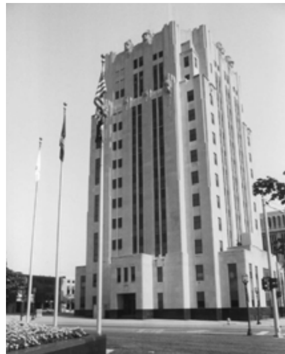
Macomb County Building 1
